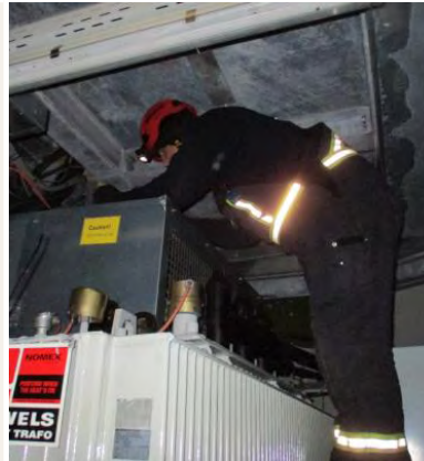
Working on Transformer
