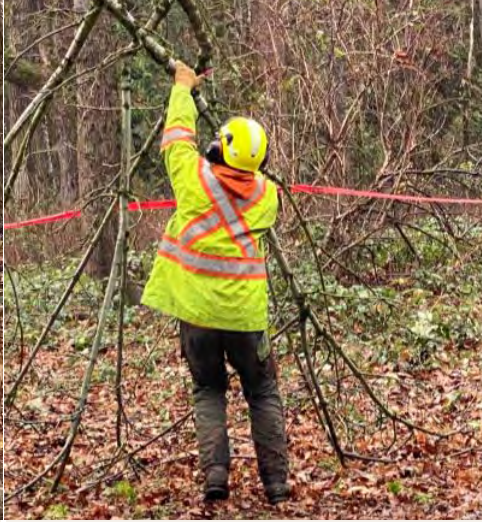
Removing rigging ropes
