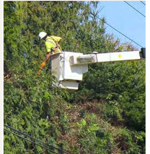
Working out of aerial lift
