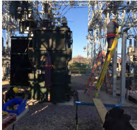
Working below ground and at heights
