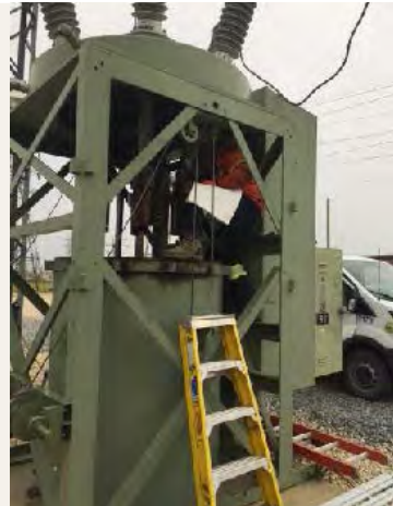
Testing and repairing equipment
