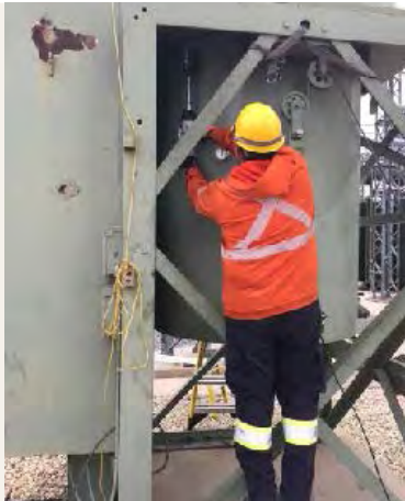
Installation of equipment
