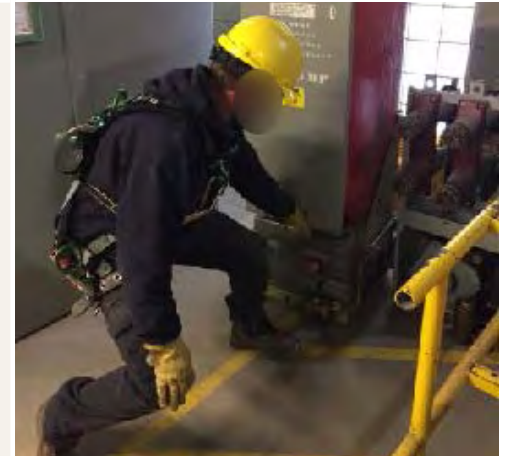
Handling of a breaker
