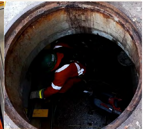
Working in confined space
