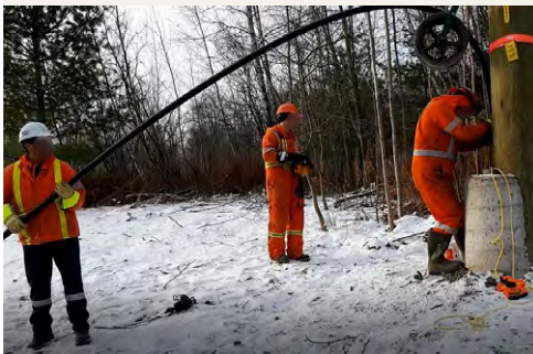
Install pulley line
