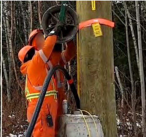
Install pulley line – 2 person lift
