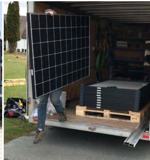
Carrying solar panel from trailer
