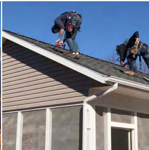
Installing roof mounts (foreground) and sounding with hammer (background)
