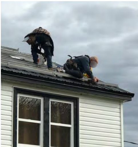
Leveling a section of rail
