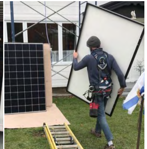
Carrying a solar panel to scaffold
