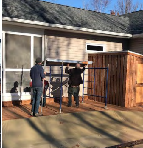
Lifting scaffold platform and positioning into place across frame members
