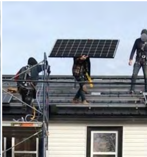
Carrying a solar panel on roof
