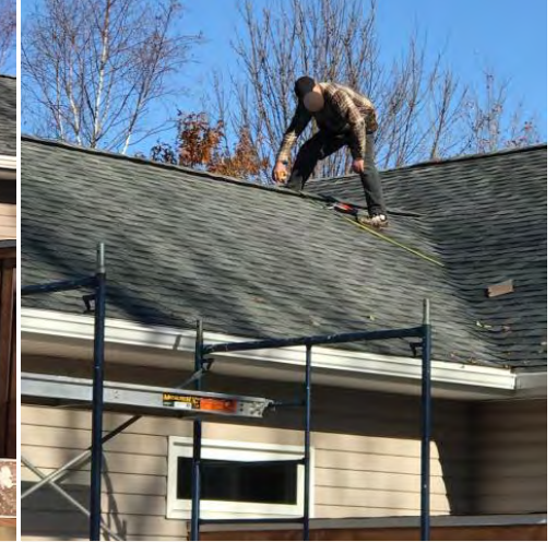
Measuring portion of roof
