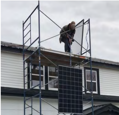
Lifting a solar panel to top of scaffolding
