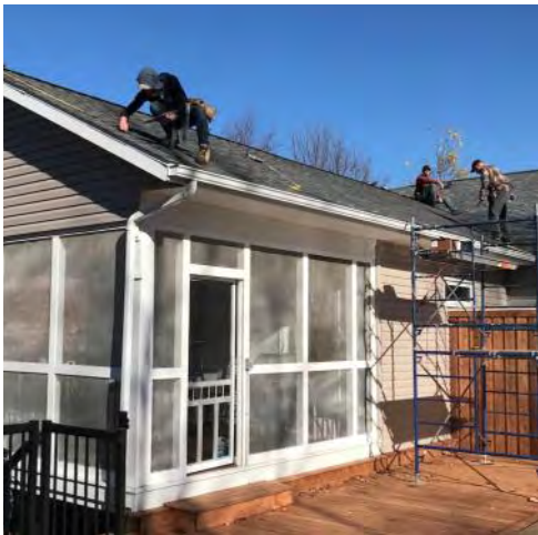
Measuring portion of roof
