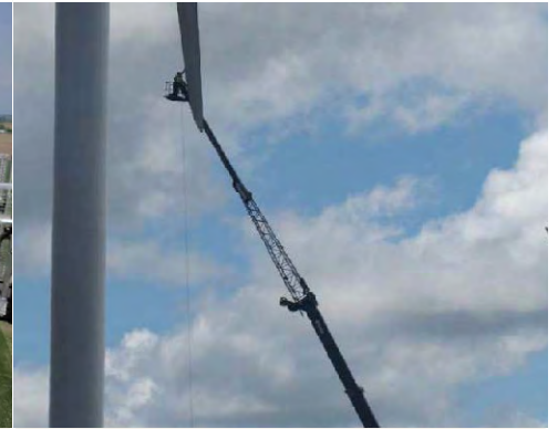
Access via crane basket
