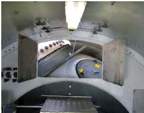
Internal access via hatches
